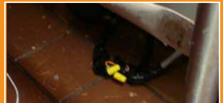
Live electrical wires expose employees to the possibility of electrical shock and increase the chance of a fire in the drive-in. These wires posed extra dangers because they were lying on a wet floor.
