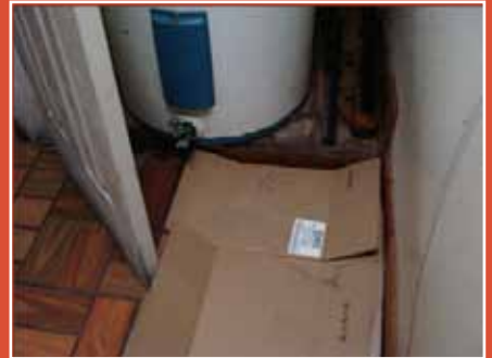
Flammables and combustibles cannot be stored with 36" of an ignition source such as a gas hot water heater.
