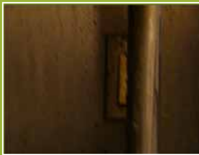
Greasy walls and electrical outlets behind warming and fryer tables will increase the chances of a fire.
