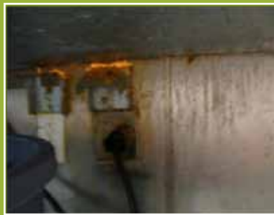
Greasy walls and electrical outlets behind warming and fryer tables will increase the chances of a fire.
