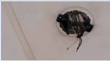
Exposed electrical wires are especially dangerous to persons and property, but can be easily corrected.
